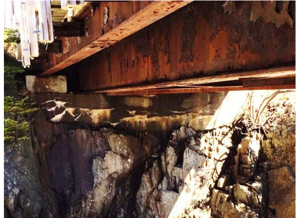
Figure 10: Abutment (Bridge 2)
