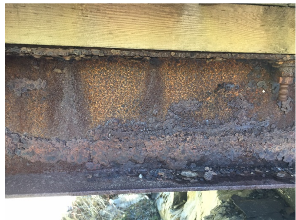
Figure 12: Deteriorated Steel (Bridge 2)
