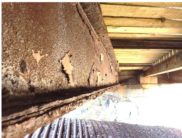
Figure 11: Deteriorated Steel (Bridge 1)
