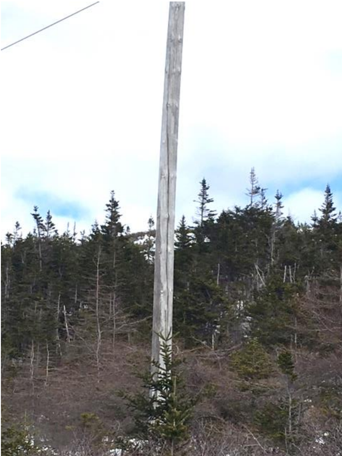
Figure 9: Significant Checks in Pole
