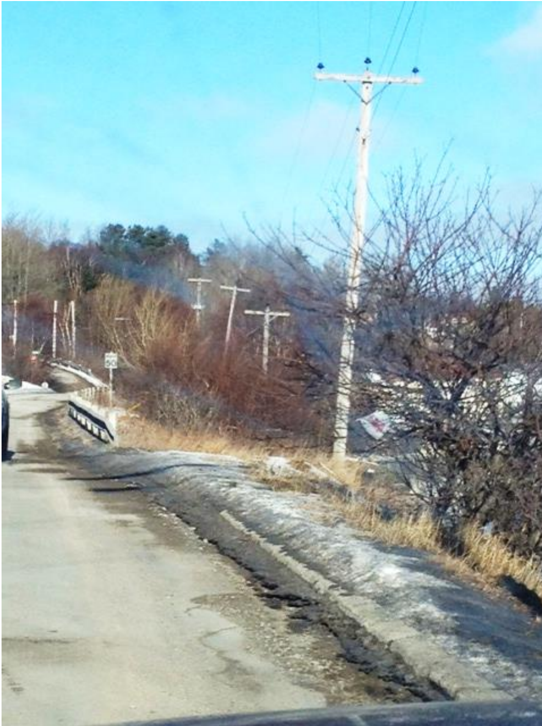
Figure 2: Deteriorated Section (Poles Leaning)
