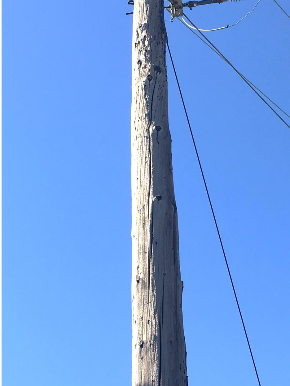
Figure 14: Deteriorated Pole with Checks
