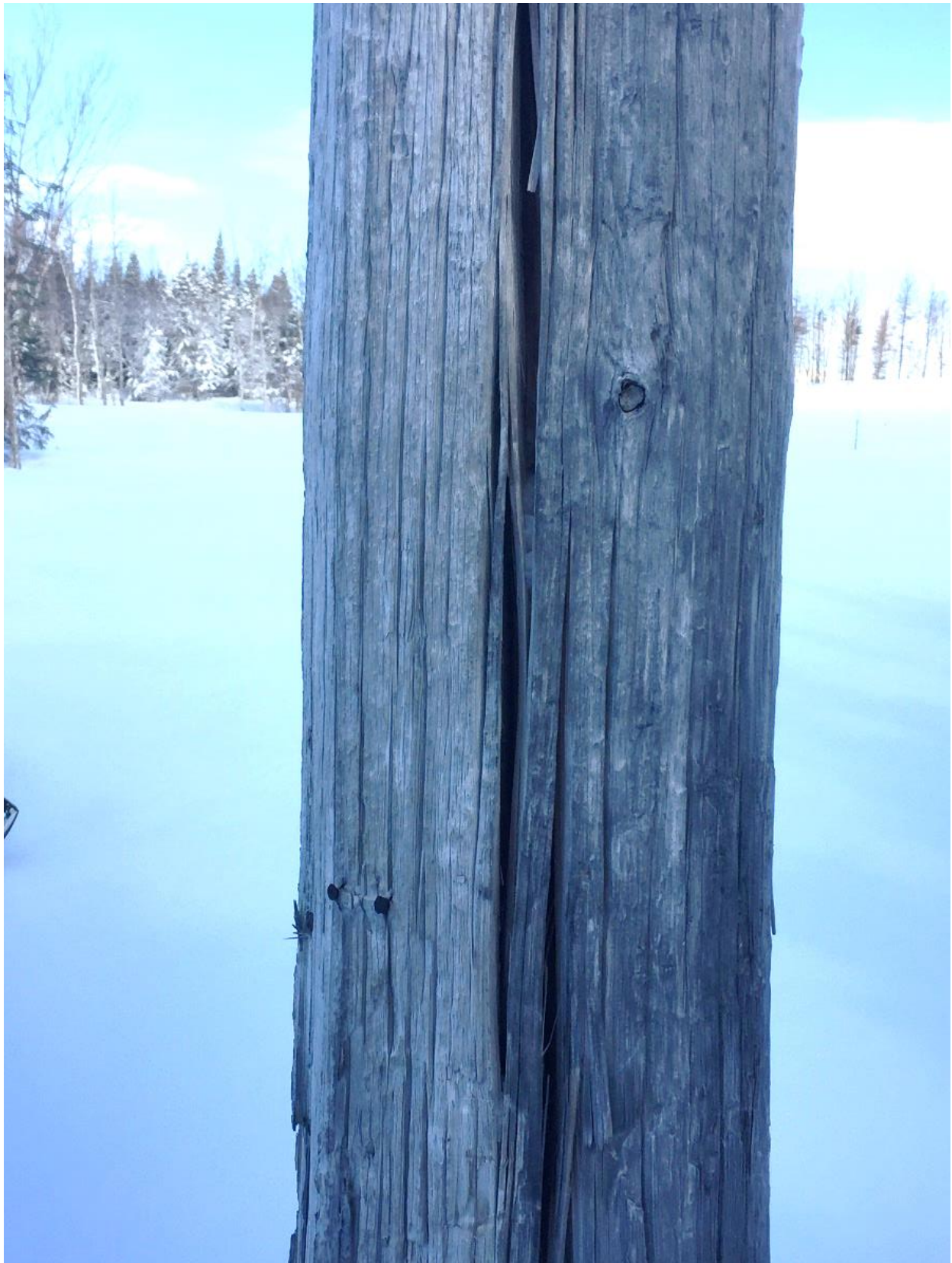
Figure 4: Severe Checks in Pole
