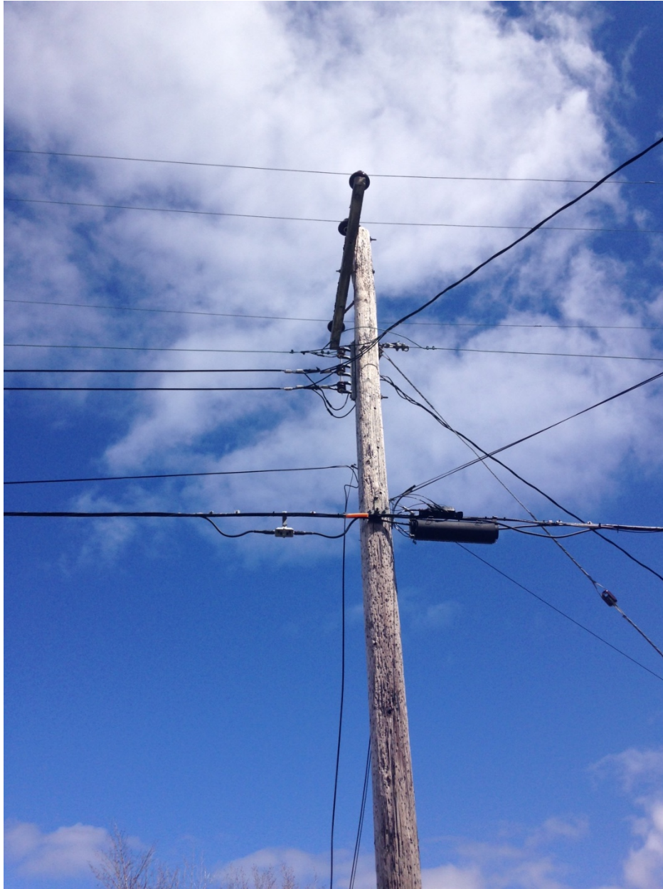
Figure 8: Non-Standard Secondary/Deteriorated Structure
