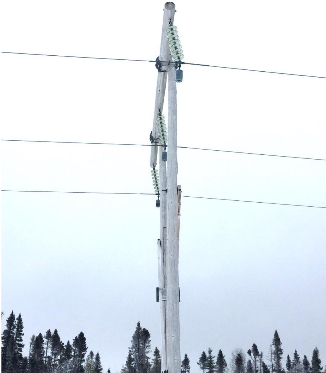
Figure 3: Structure Twisted as a Result of Storm Loading
