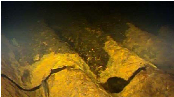
Figure 7: Cracked and Corroded Section
