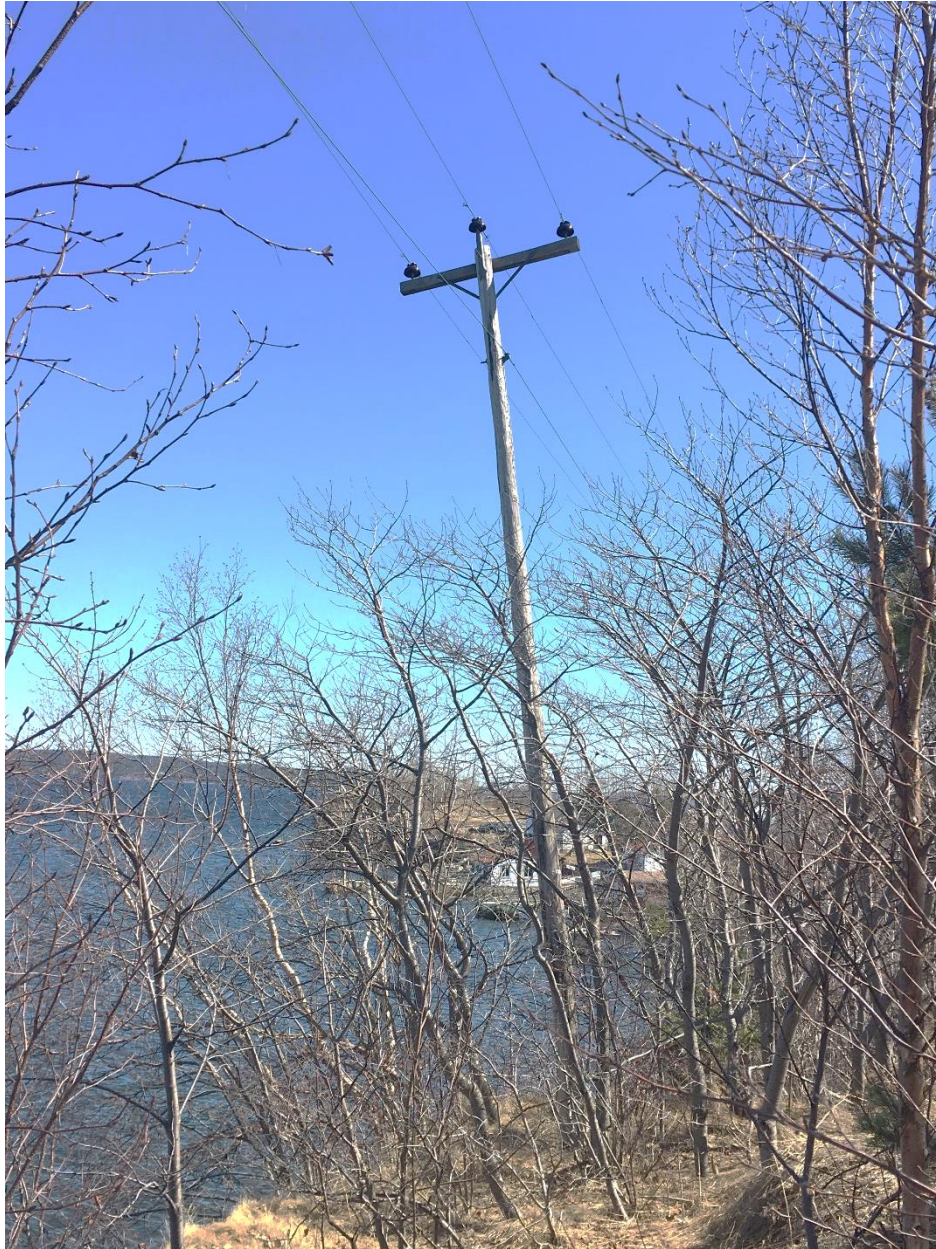
Figure 11: Deteriorated Leaning Pole
