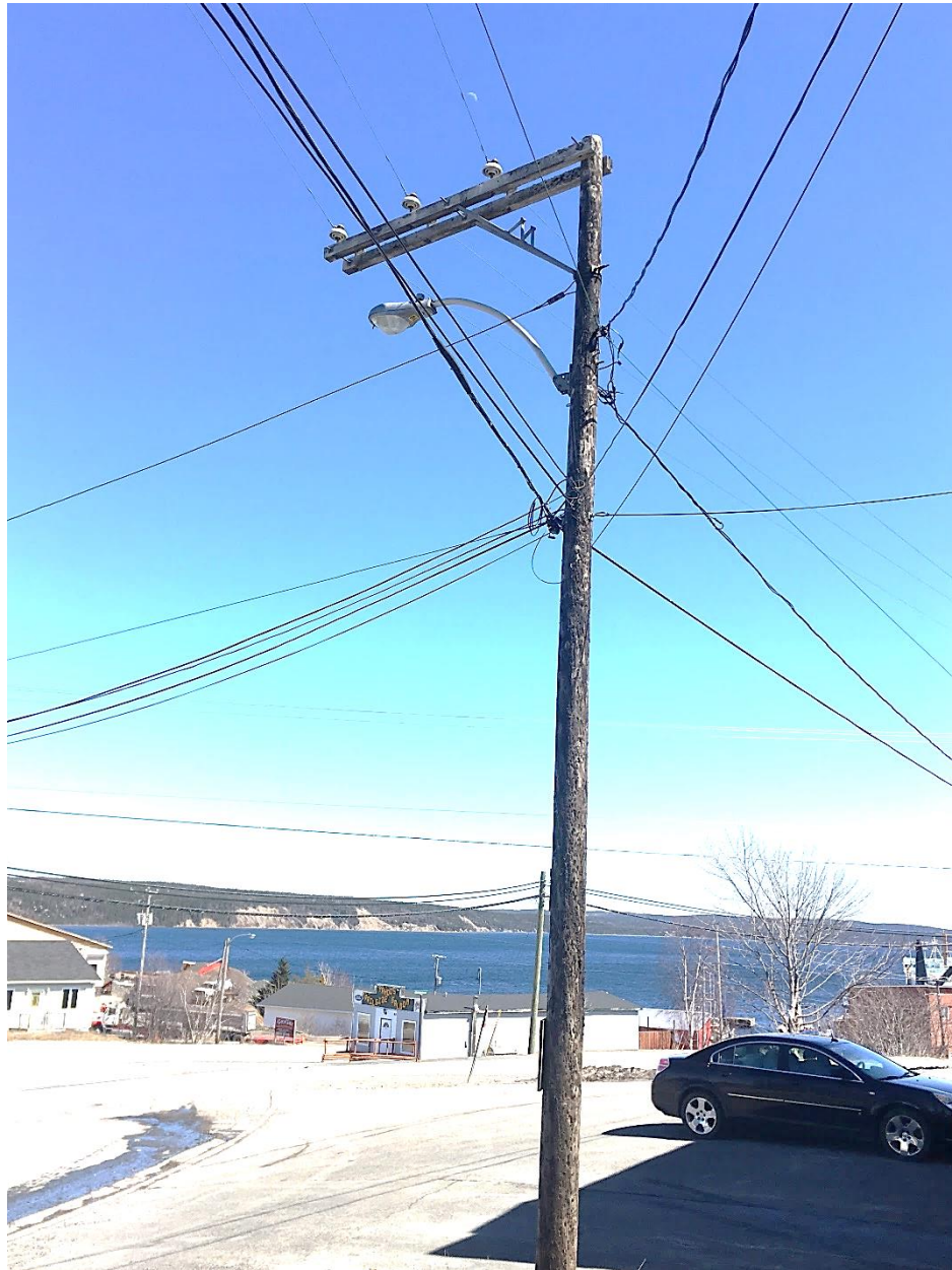
Figure 9: Non-Standard Construction/Substandard Clearances
