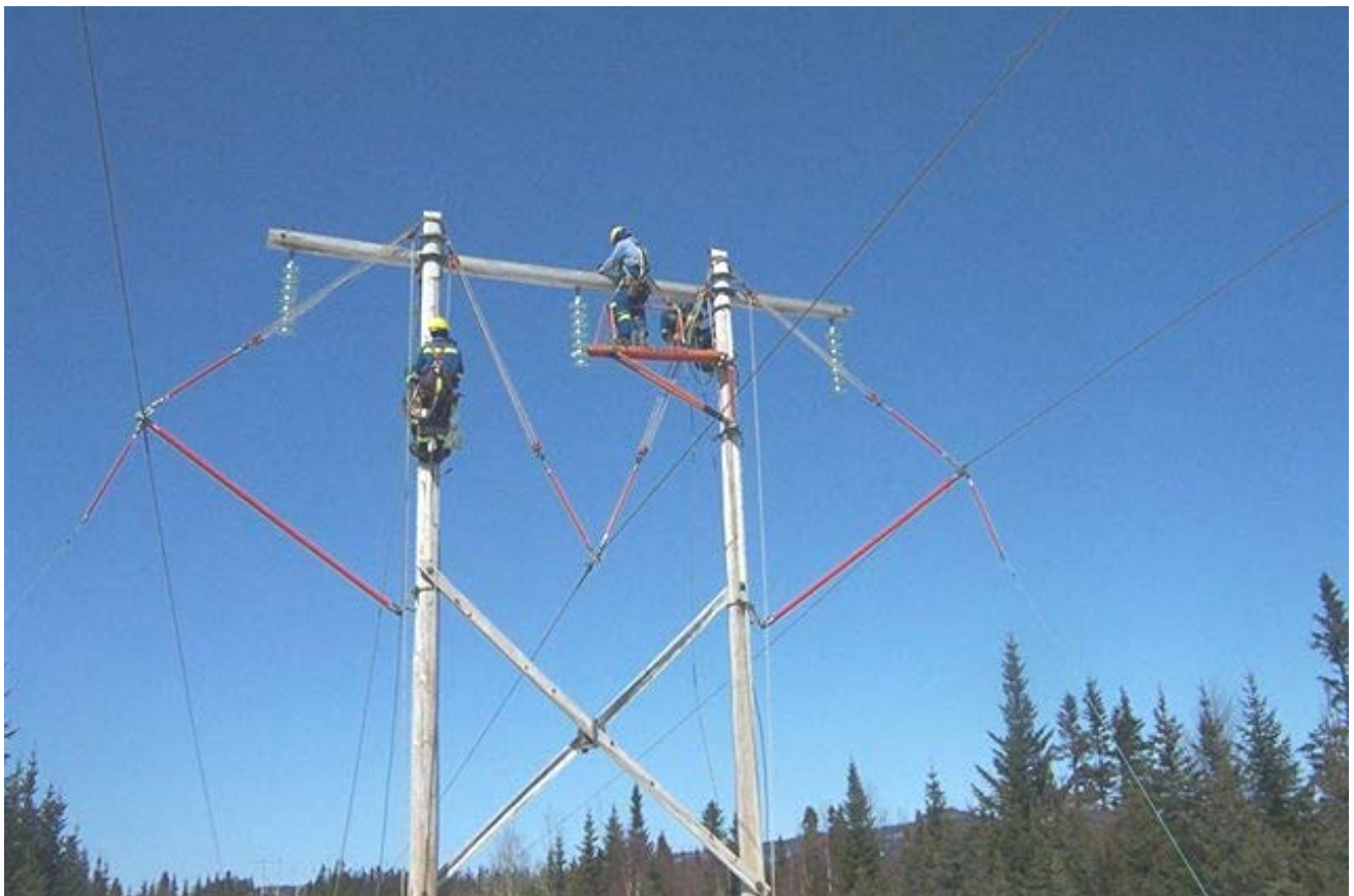
Figure 8: Replacement of Insulators on 363L Using Hot-Line Work Method
