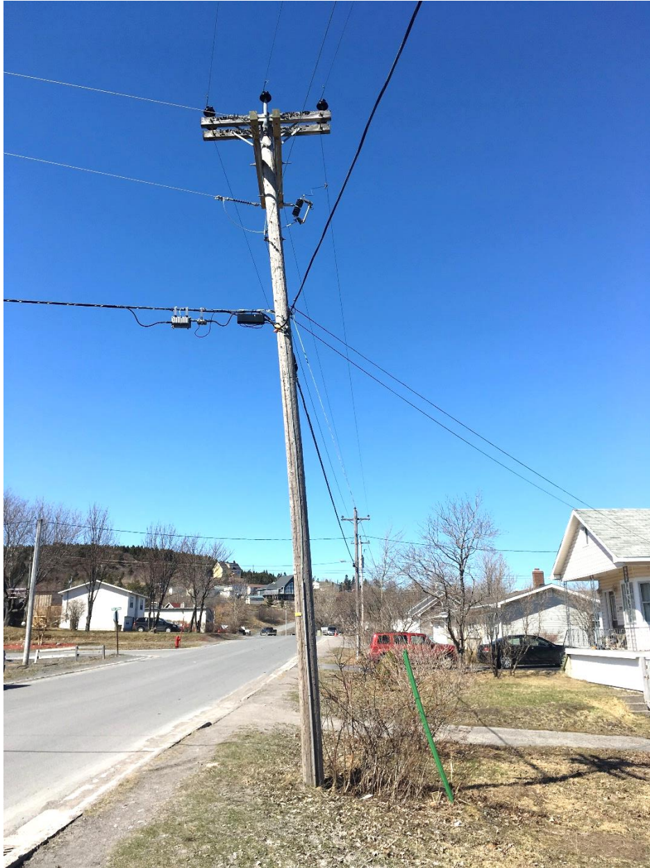
Figure 15: Leaning Non-Standard Structure
