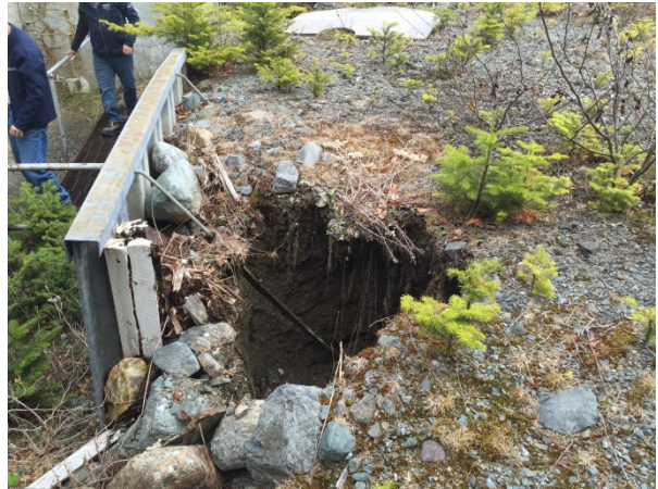
Figure 6: Right Side Sinkhole
