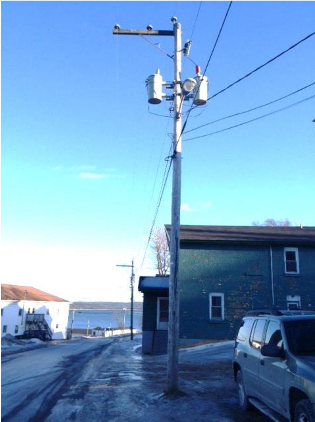
Figure 6: Deteriorated Line/Substandard Clearances
