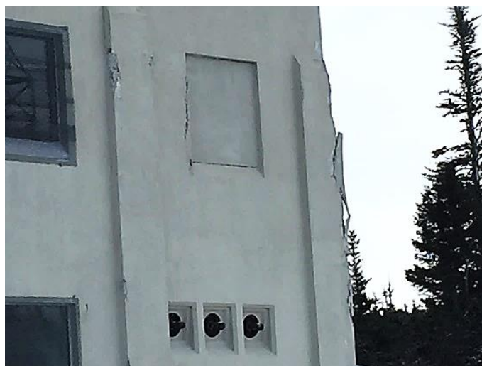
Figure 15: Powerhouse Parging Failure
