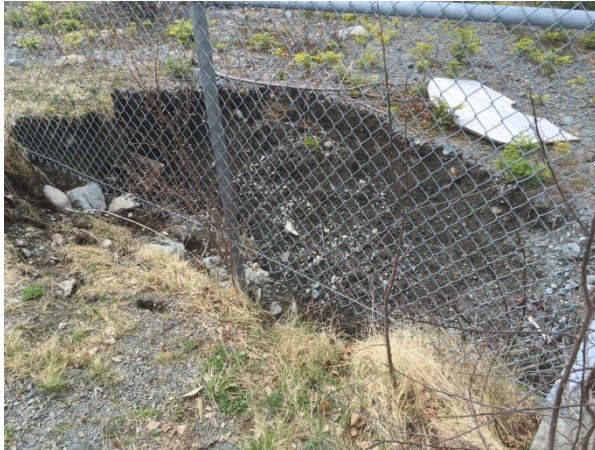
Figure 5: Left Side Sinkhole
