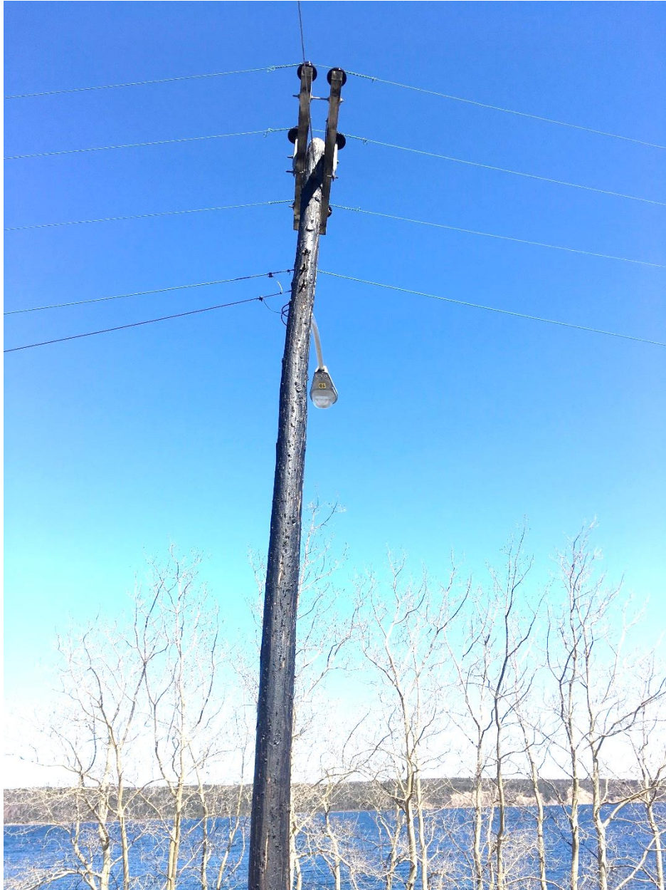
Figure 10: Deteriorated Leaning Pole
