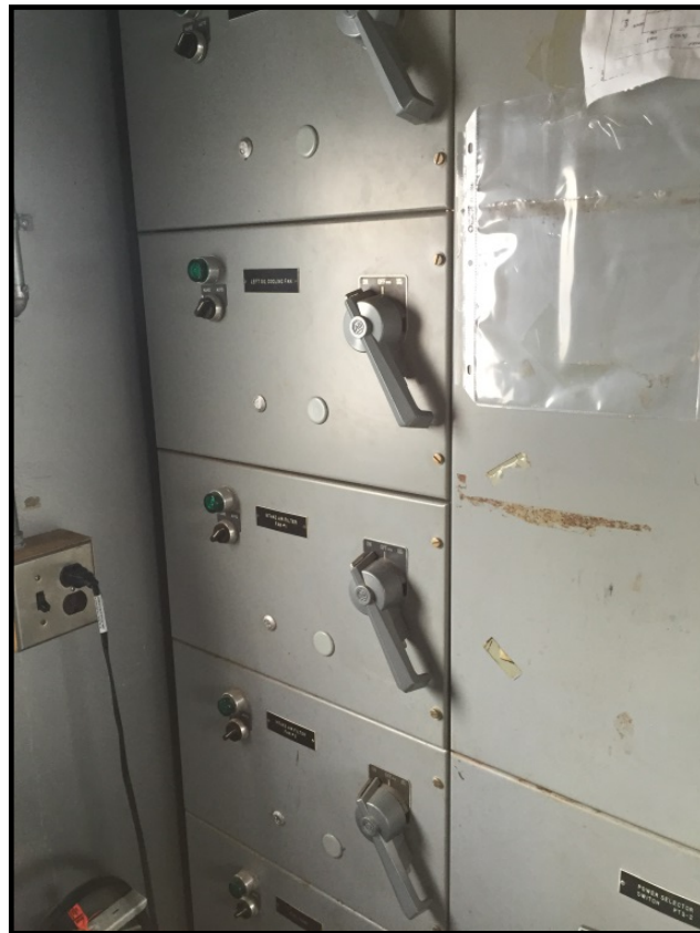
Picture 12: Motor Control Center
