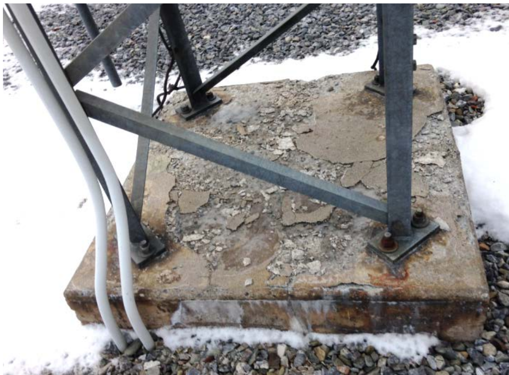
Figure 7: BVS Deteriorated Concrete Foundation
