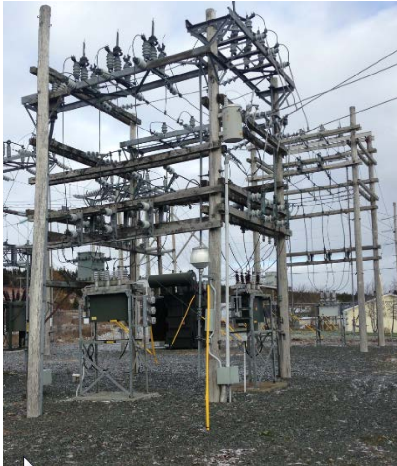
Figure 4: HGR Hydraulic Reclosers
