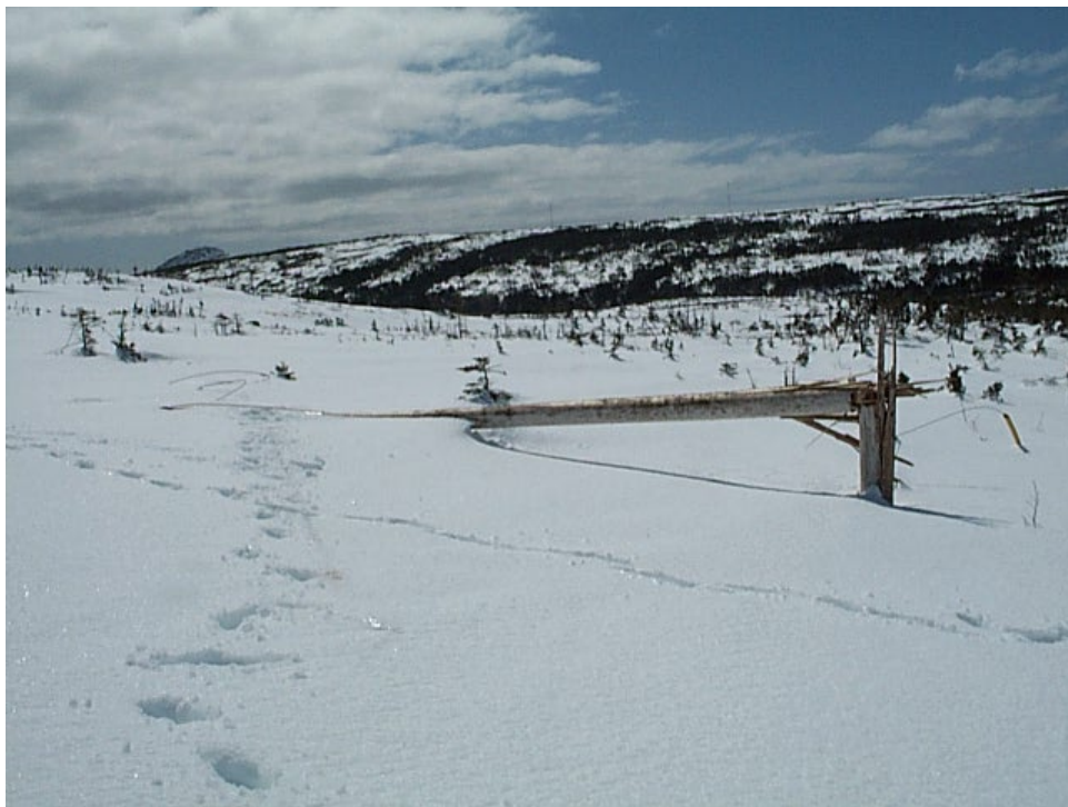
Figure 12: Line Failure During Severe Icing Event
