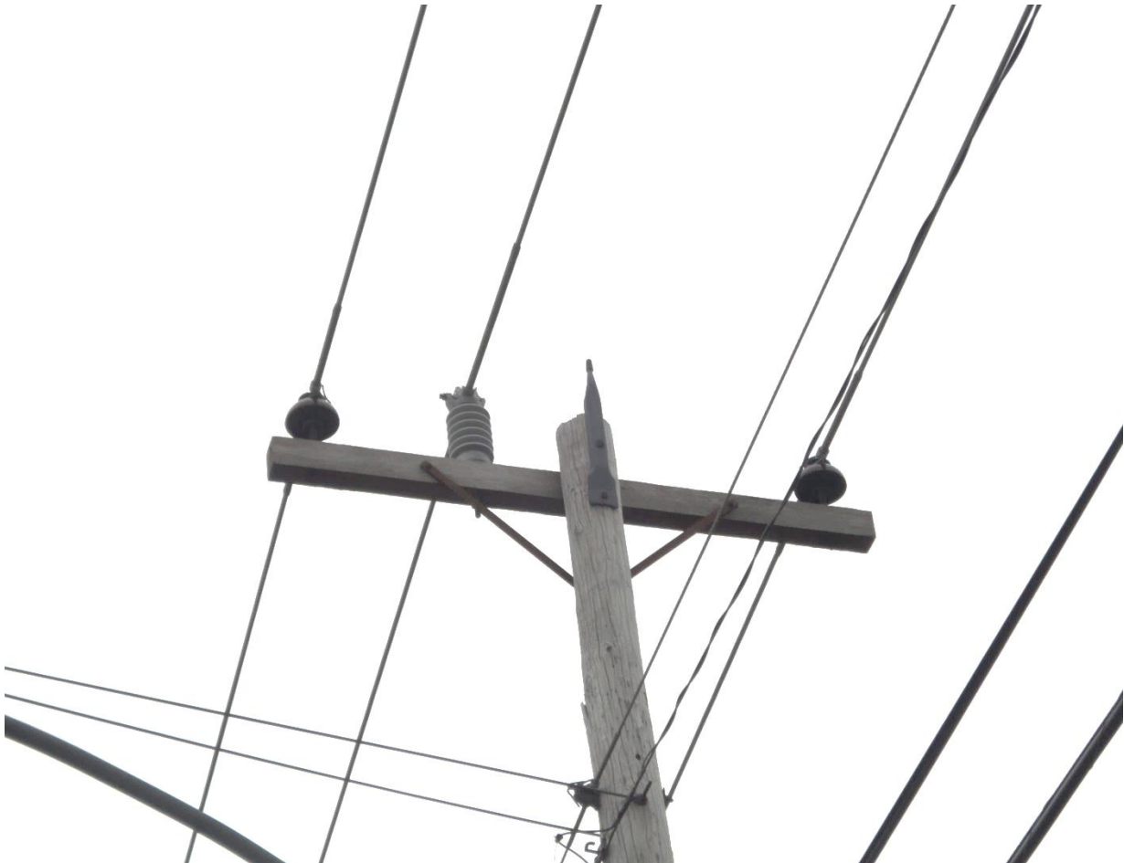
Figure 3 – Previously Failed 2-Piece Insulator
