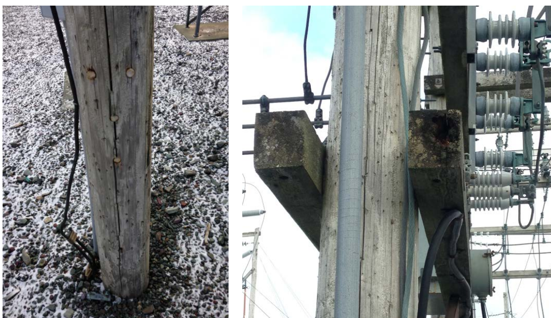
Figure 2: HGR Deteriorated Wood Poles and Cross Arms
