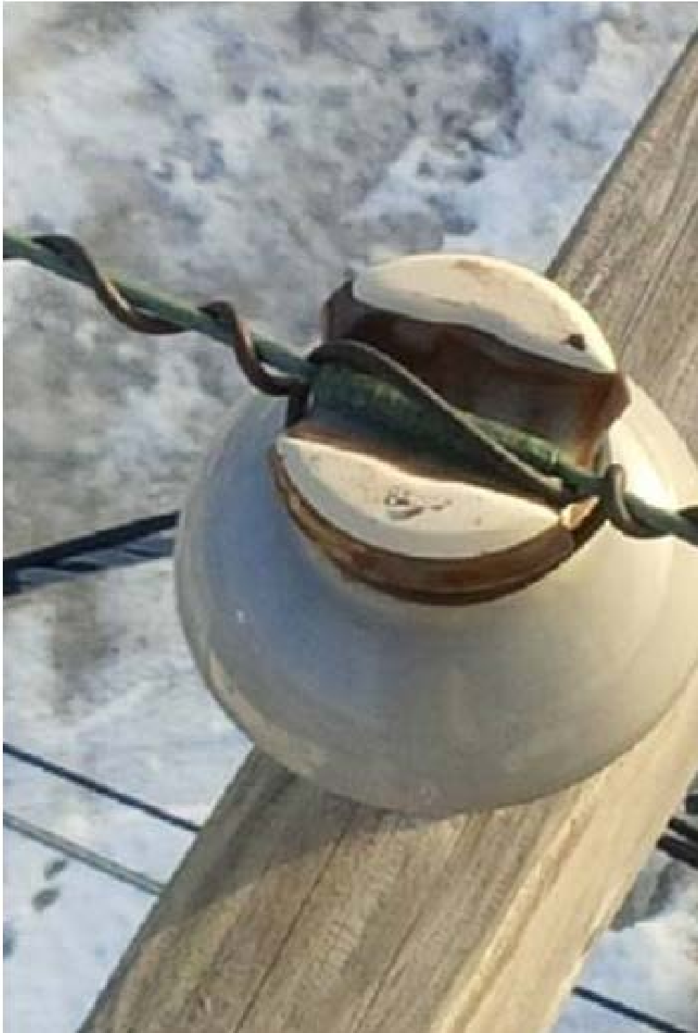
Figure 5: Hidden Splice on Insulator (Potential Hazard)
