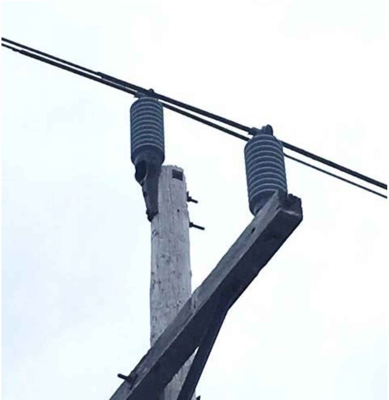
Figure 10: Decay at End of Wooden Crossarm
