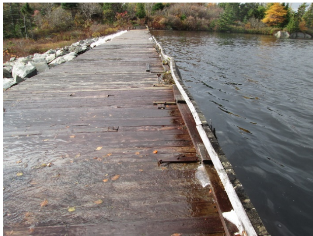
Figure 3: Misaligned Upstream Face
