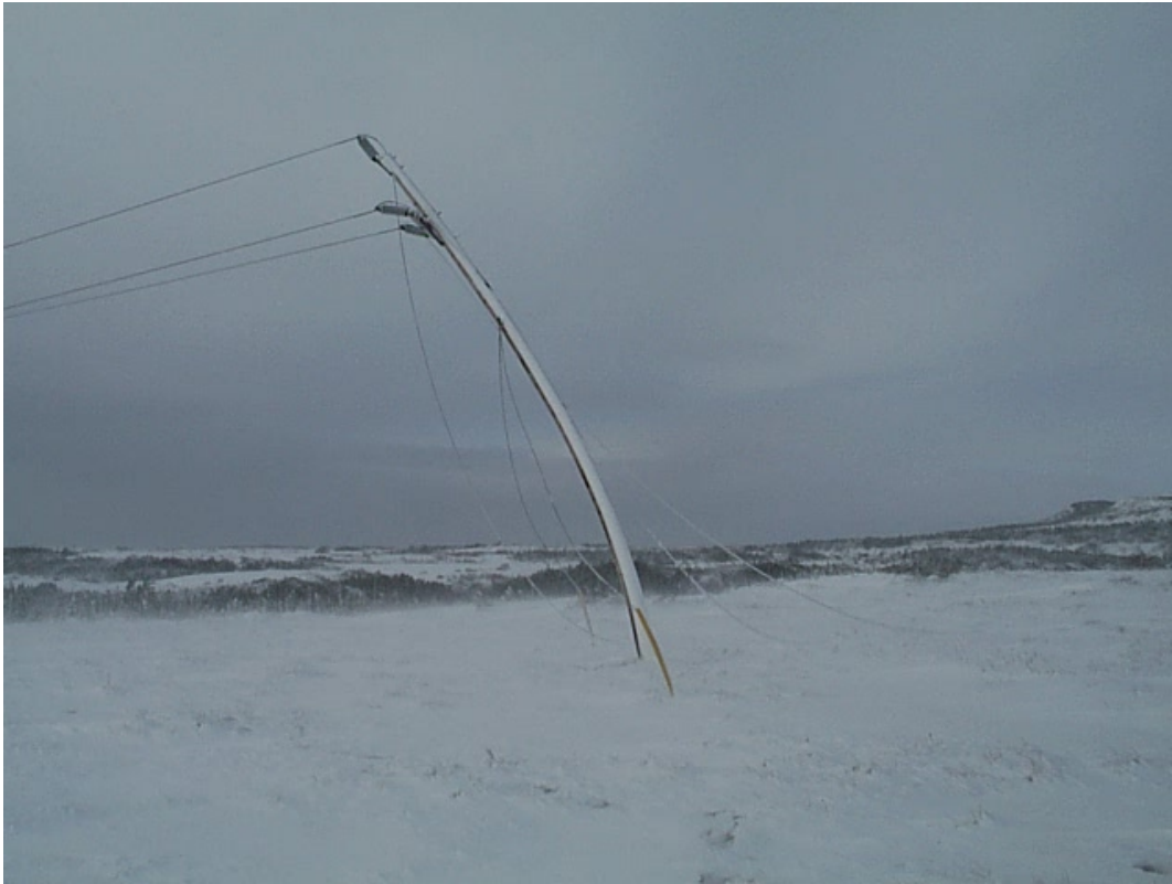
Figure 11: Structure Damage Due to Conductor Failure
