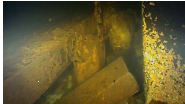
Figure 8: Failed Culvert to Concrete Connection
