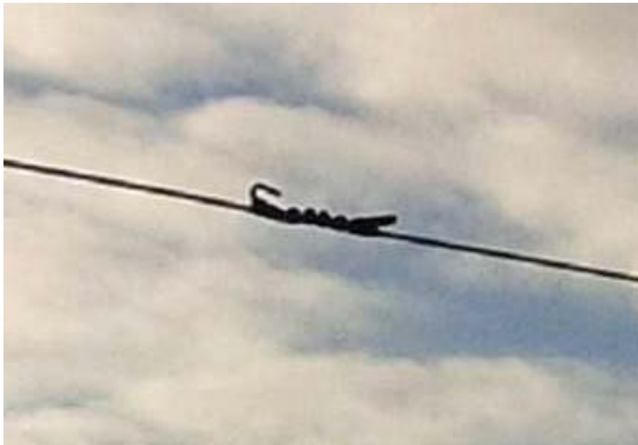
Figure 4: Splice in #4 Copper Primary Conductor
