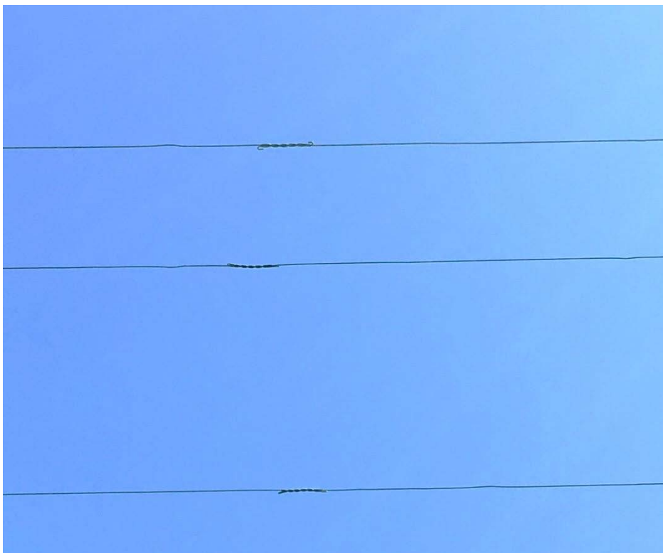
Figure 13: 3 Splices in #4 Copper Primary Conductor
