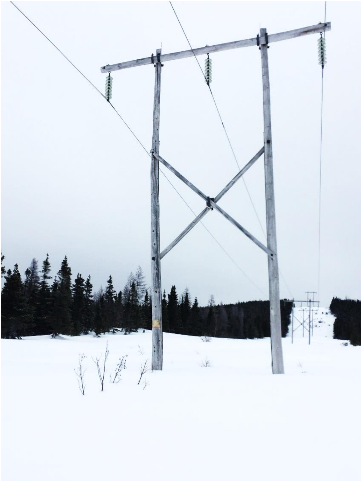
Figure 1: Check in Left Pole Near Crossbrace Attachment
