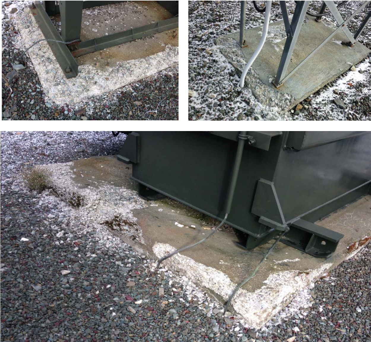
Figure 3: HGR Deteriorated Concrete Foundations
